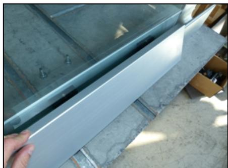
The Rail covers are pre-fitted with 3M tape. Cut Cover to size allowing for any corners or mitred cut outs. Please ensure main channel is clean and free from debris or grease. Remove 3M backing tape and carefully position the cover by engaging the top section first and then slowly lowering the sides down. This ensures cover is correctly engaged on the top of the channel.
