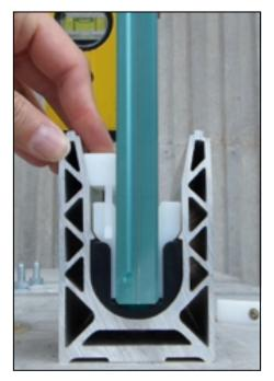
Once glass is in place insert one clamp wedge in position. Using a spirit level against the glass slowly press the clamp wedge down until the bubble is central. If you press down too much raise and repeat process.
