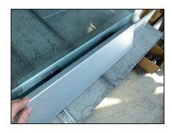
The Rail covers are pre-fitted with 3M tape. Cut Cover to size allowing for any corners or mitred cut outs. Please ensure main channel is clean and free from debris or grease. Remove 3M backing tape and carefully position the cover by engaging the top section first and then slowly lowering the sides down. This ensures cover is correctly engaged on the top of the channel.
